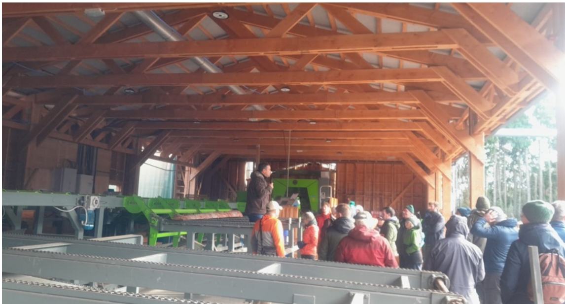
Photo 12: Newly commissioned mill. Roof was constructed using all Scottish timber.
